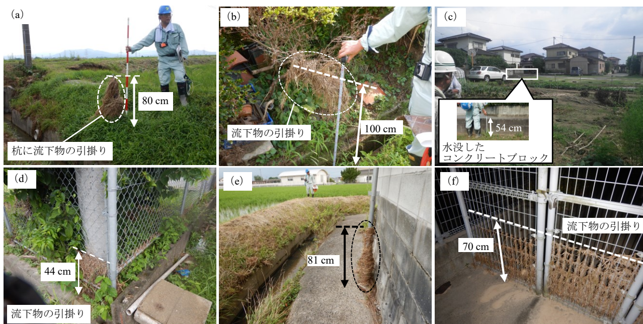
Fig. 4 氾濫域の浸水痕跡 Flood trace due to Nakashima-ike dam breach
